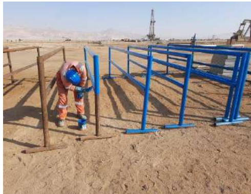
Fabricated Handrail for Roads
