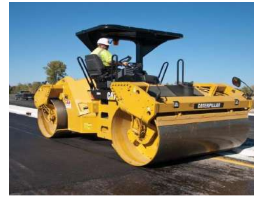
Soil and road leveling works for Rigs
