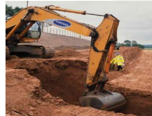
Excavation and filling Contracting
